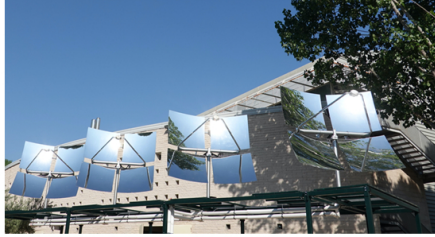
Small dishes put up by Spanish company TCT – Thermal Cooling Technology at a sports centre near Madrid Photo: TCT
